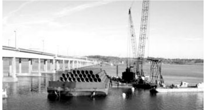
Wilson Bridge pile-driving operation on the Potomac River.
