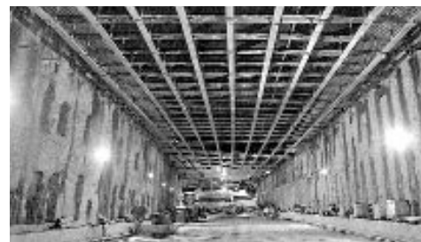
Tunnel construction on the Central Artery/Tunnel Project in Boston.
