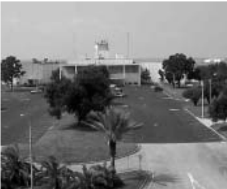
New Orleans Lakefront Airport, Terminal Building, New Orleans, LA
