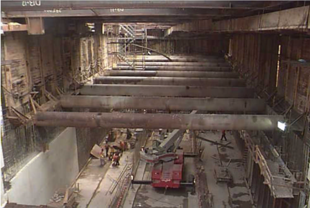
Figure 1. Construction at the Universidad Station in Rio Piedras.
