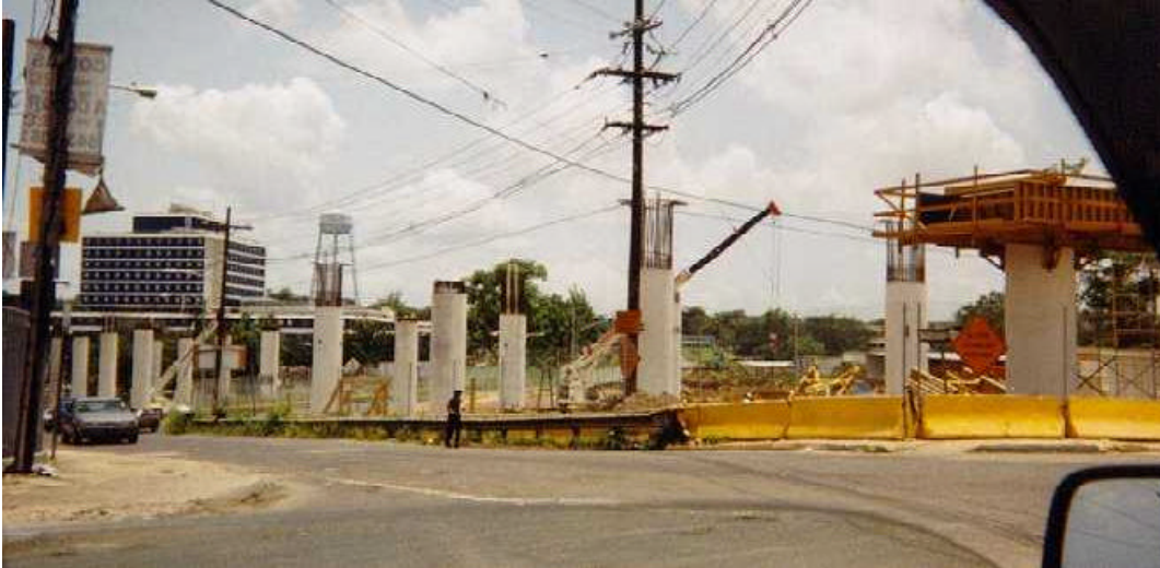
Figure 2. Construction of Columns on the Tren Urbano
