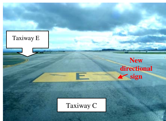
Figure 3. Surface Painted Taxiway Directional Sign at San Francisco International Airport
