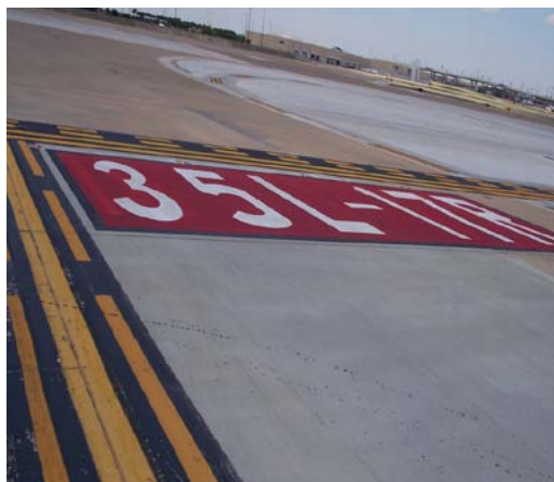
Figure 2. Enhanced Surface Markings at Dallas/Fort Worth International Airport
