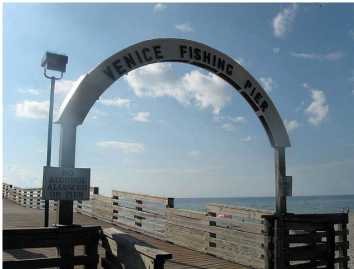
Figure 2 Access to the fishing pier is integrated into Sharkey's on the Pier's leasehold.
