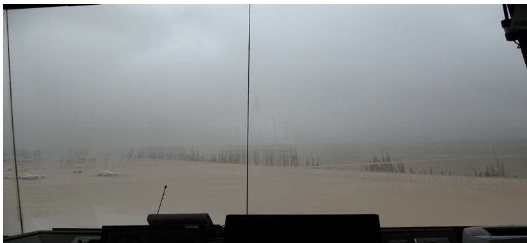
Figure 3. Condensation on Tower Windows at Andrews ATCT Hinders Air Traffic Controllers’ View of the Airfield
