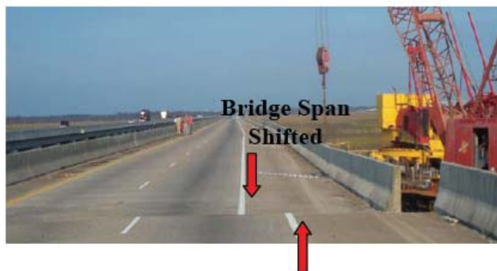
Figure 3: I-10 Bridge Repair at Pascagoula
