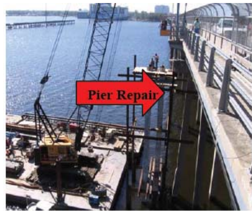
Figure 6. I-110 Bridge Repair
