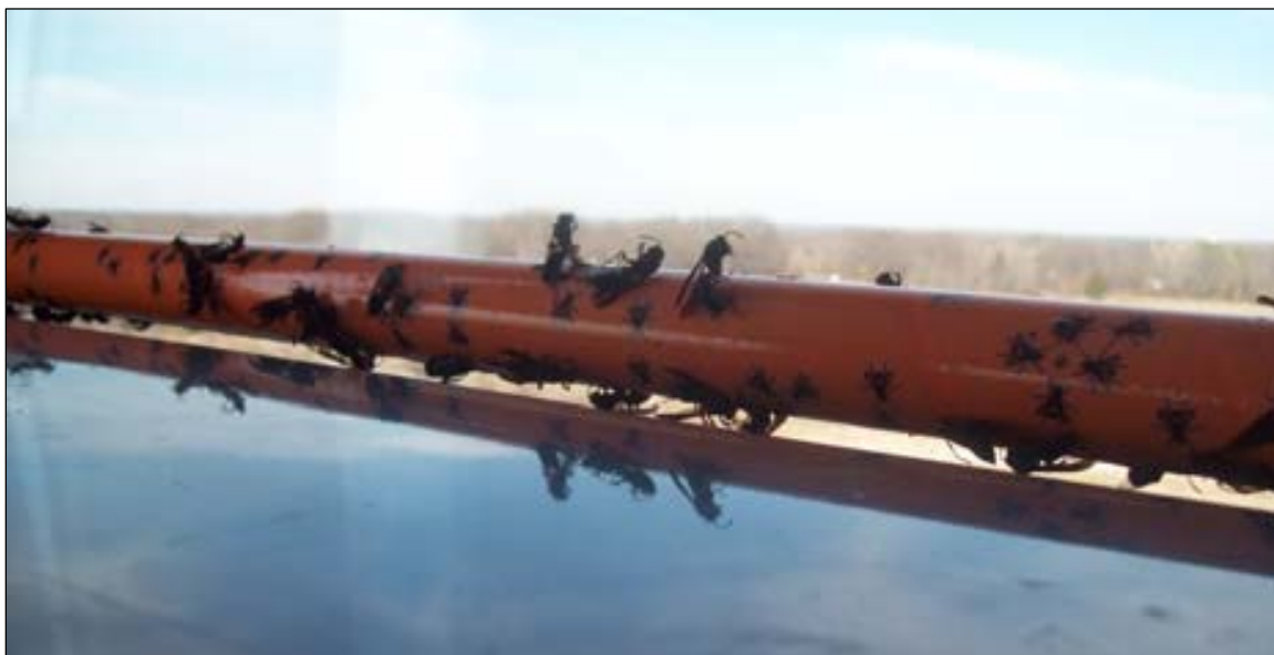
Figure 3. Wasp Infestation Inside Airport Tower
